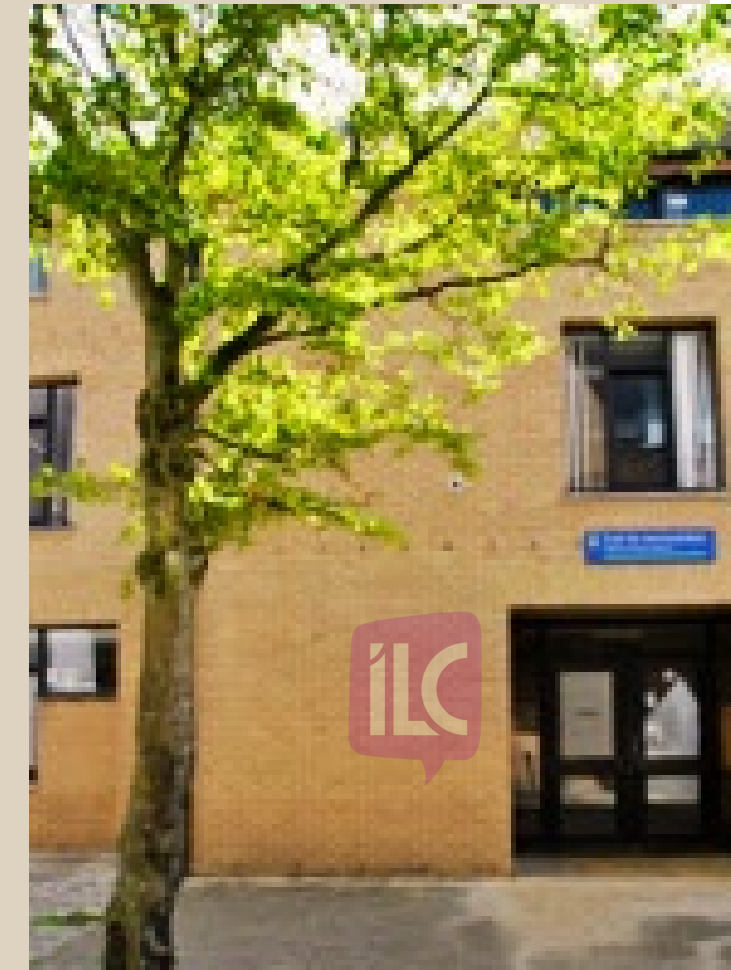
Also in DUPRIEZ BUILDING GROUND FLOOR local E.012
